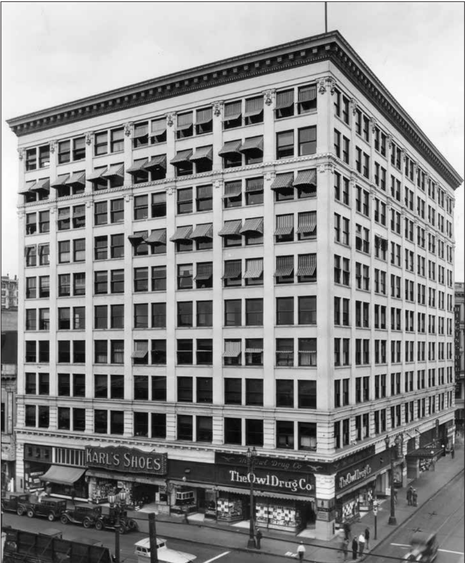
Figures 18–19. Above: The Higgins Building (1910), designed by A. L. Haley, with A. C. Martin as structural engineer, was an early monument to reinforced concrete technology. Originally planned as an eight-story building to meet local height restrictions, Haley won approval to extend the structure to ten stories. Notice the string course marking off the added two stories in this 1941 photograph. See also the architect’s rendering in Figure 6. Art Streib, Herald Examiner Collection , Los Angeles Public Library. 00058765. Opposite: Reinforced concrete construction: After the forms were removed from the second floor of the Higgins Building. Haley, “A Ten Story Monolithic Reinforced Concrete Building,” 39.
