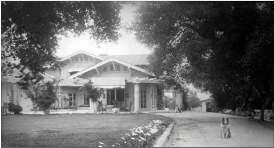
Figure 1. The Lanterman residence (1915), a Craftsman-style home of reinforced concrete in then sparsely settled La Cañada-La Crescenta Valley, was designed by architect Arthur L. Haley to be fire resistant and earthquake proof. Many of its features echo those of Haley's extensive practice in Los Angeles office and apartment design. Courtesy of the Lanterman House Archives.
