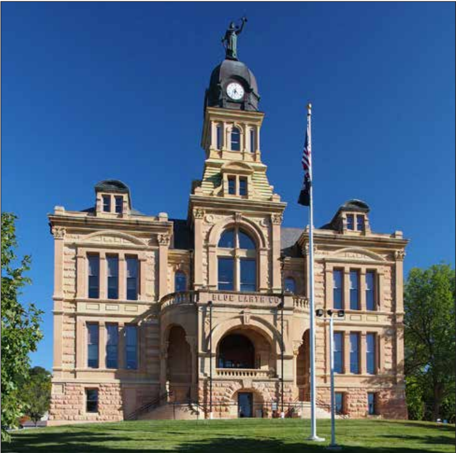
Figure 3. In his early twenties, A. L. Haley won a competition to design the Blue Earth County courthouse in Mankato, Minnesota. It was constructed between 1886 and 1889 at a cost of $200,000. It still stands today and is now on the National Register of Historic Places. File:Blue Earth County Courthouse.jpg Wikimedia Commons, 11 September 2021, 12:10 UTC, < https://commons.wikimedia.org/w/index.php?title=File:Blue_Earth_County_Courthouse.jpg&oldid=590468463 > [accessed 21 June 2023]. Photo by McGhievers, licensed under CC by 4.0.
